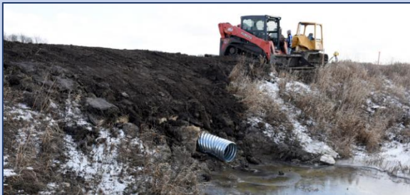
Above: Pennington County side water inlet project to reduce erosion (BWSR). Below: Turbid ditch water (RLWD)
